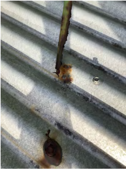
Example of rusted metal brackets on roof.
