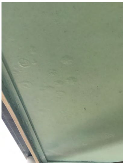
Example of blistered/bubbled paint.
