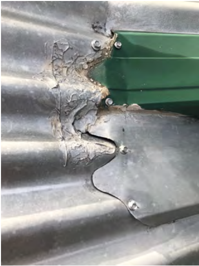
Example of poorly flashed Patio/Main roof junction.
