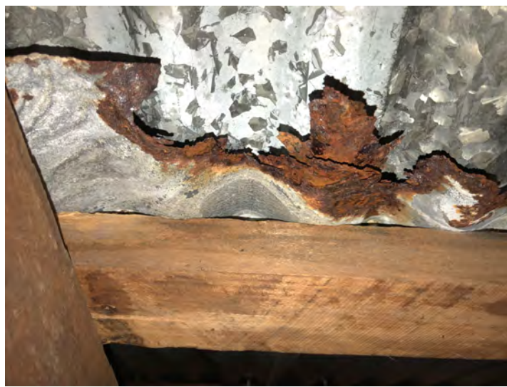
Example of rusted ends of roof sheets.
