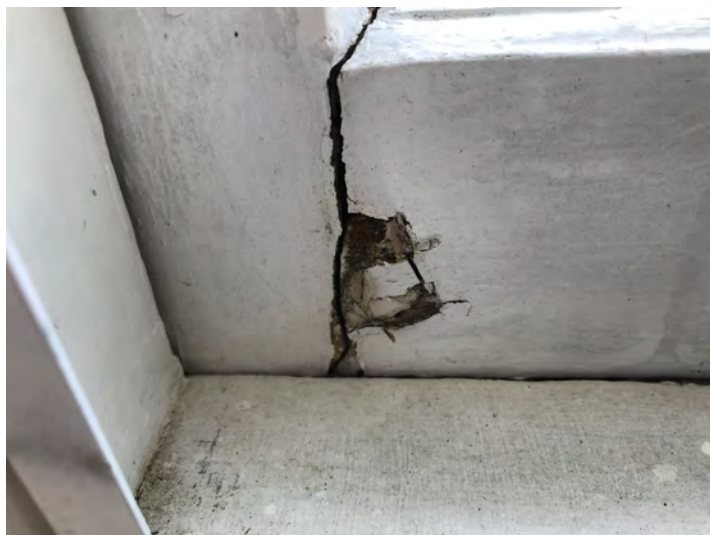
Example of Wood Rot to timber window.
