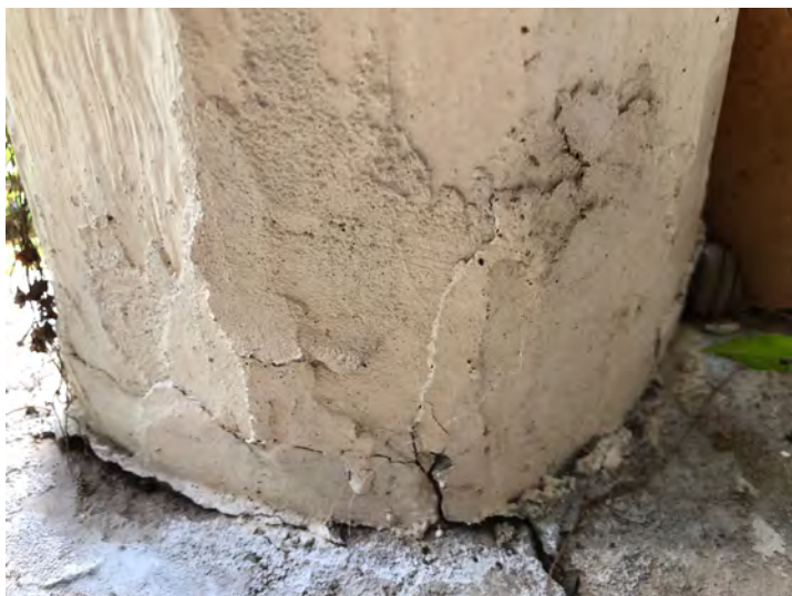
Example of House post bases encased in concrete/mortar.
