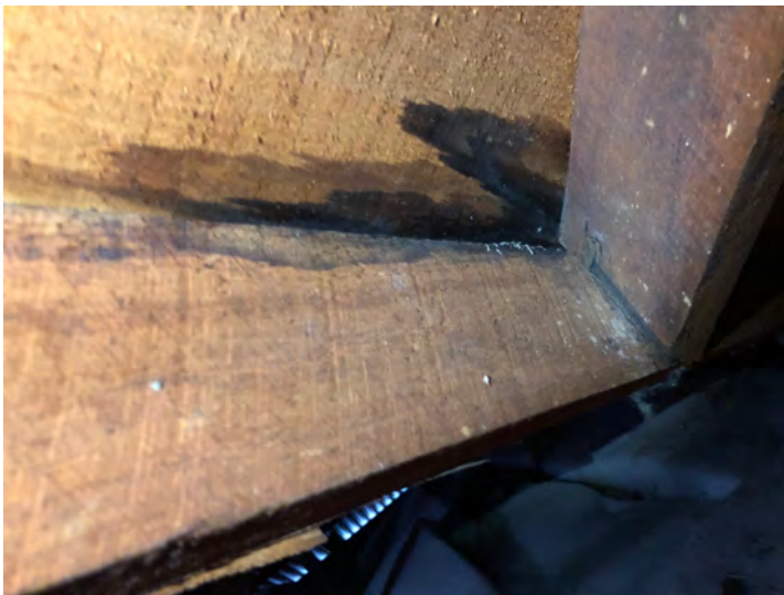
Example of water staining/leaks into roof space below rusted valley gutter.
