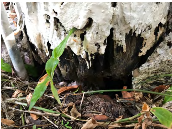
Example of deteriorated/ pencil pointed bases of posts.
