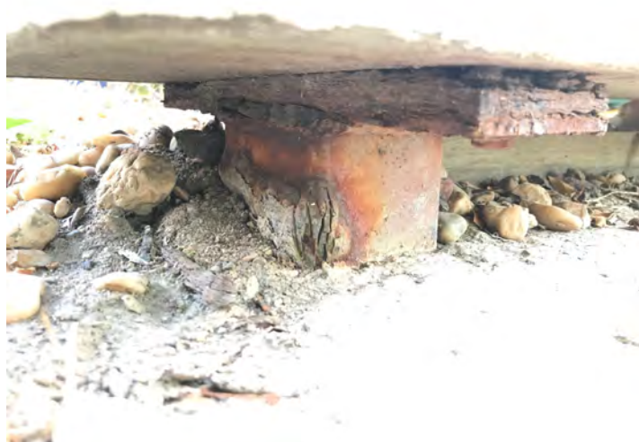
Example of rusted steel posts under stairs.
