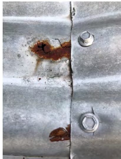
Example of rusted laps/joins to roof sheeting.
