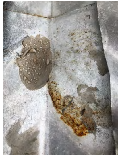
Example of rusted laps/joins to one or two valley gutters.
