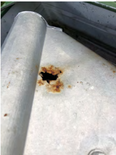
Example of rusted parts to ridge cappings.
