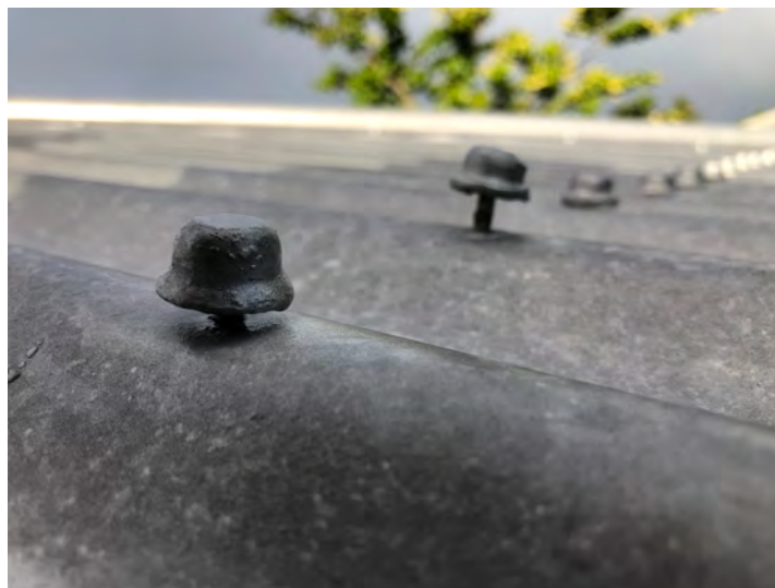
Example of loose nails.
