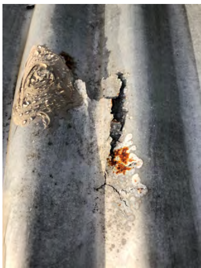
Example of rusted laps/joins to roof sheeting.
