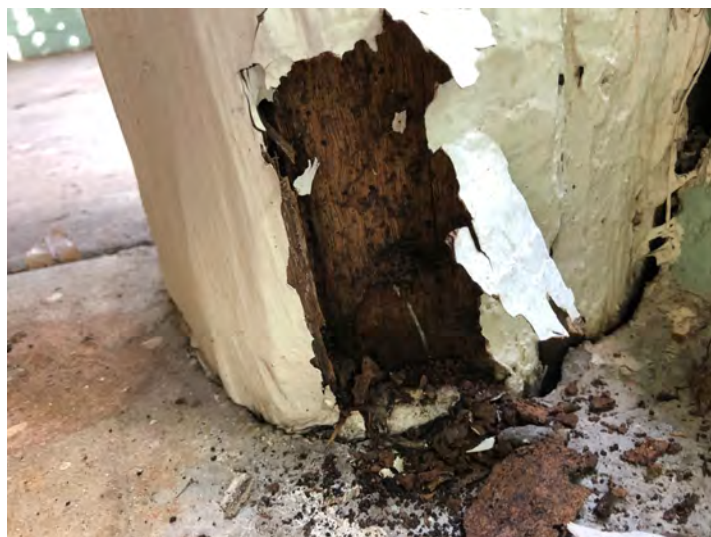
Example of Termite damaged House post.
