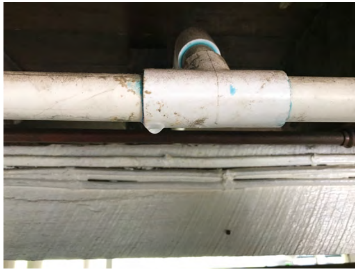
Example of leaking water pipe.
