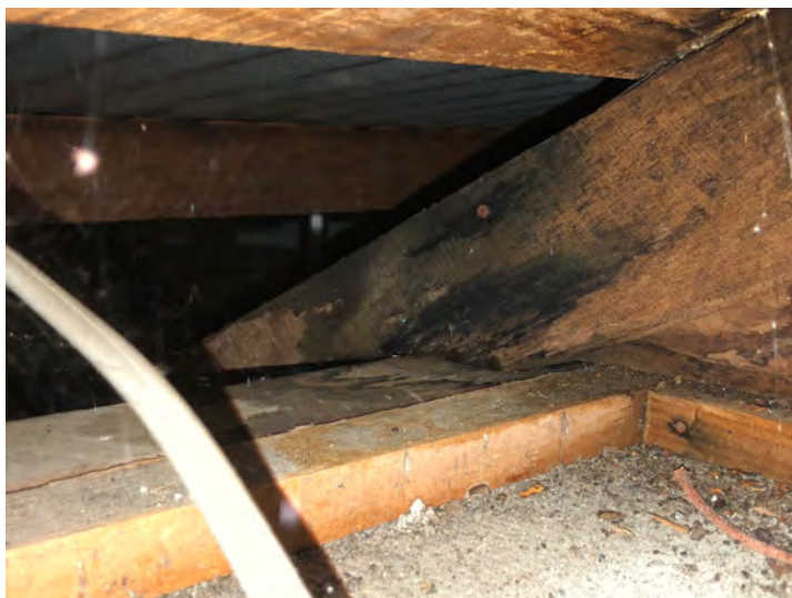
Example of water staining/leaks into roof space.
