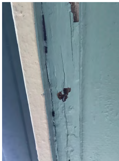
Example of water damaged soffit moulding.
