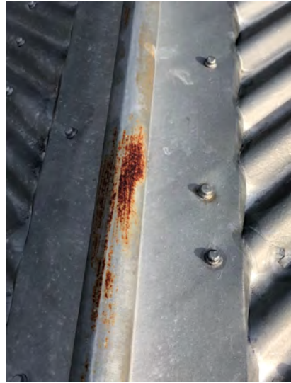
Example of rusty parts to ridge cappings.
