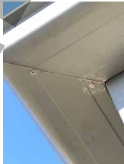
Example of corrosion starting to parts of gutters.
