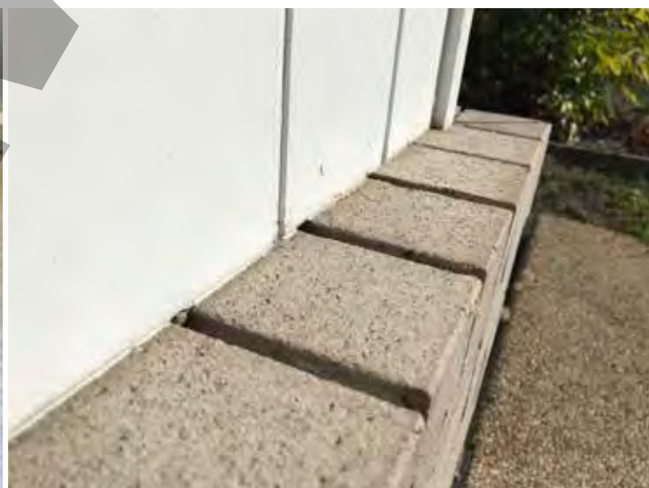
Example of no flashing installed at front.
